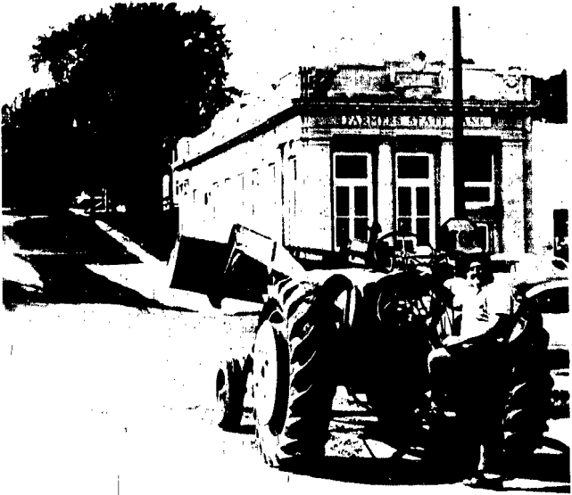
CARROLL STREETS are getting new armor coating Mayor Perry Johnson helps out with the work. He was stopped just long enough to get his picture Thursday. Some of the surfacing work can be seen on the left side of the picture.
